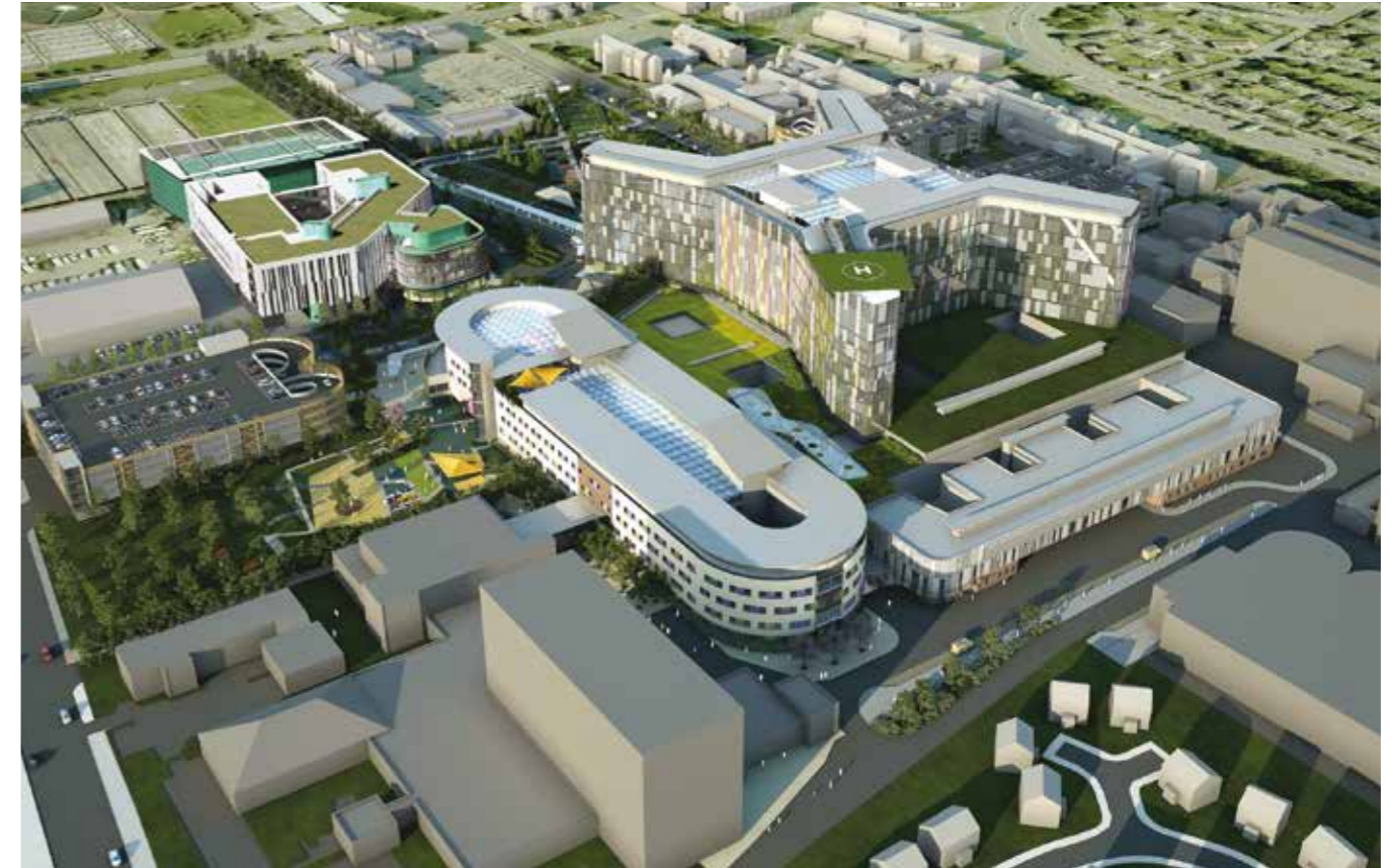
Proje: New South Glasgow Hastane Projesi / Project: New South Glasgow Hospital Project
